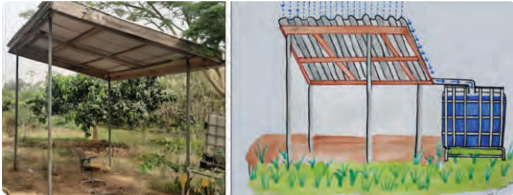
Figure 63: A small, low-cost rooftop water harvesting structure can be constructed on a farm to collect rainwater for irrigation.
