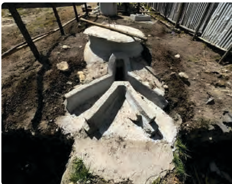
Figure 77: SAA-Ethiopia constructed two biogas chambers at farmers' houses as part of the Urban Agriculture Initiative in Lemi Kura sub-city, Addis Ababa. This initiative was supported by Ethiopia's Ministry of Water and Energy and the National Biogas Program Coordination Unit (NBPCU).
